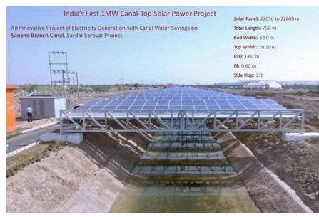
Figure 42 Solar power over Narmada canal
