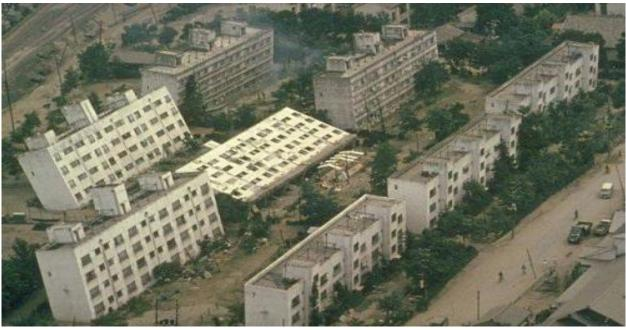
Figure 46 Effect of Soil Liquefaction
